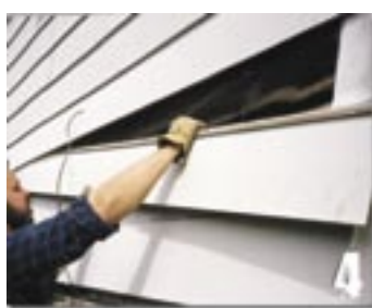
Siding carefully replaced.
