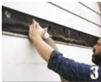
Applegate Insulation® installed.
