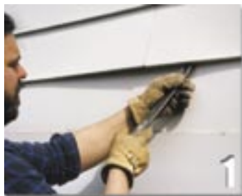
Siding carefully removed.
